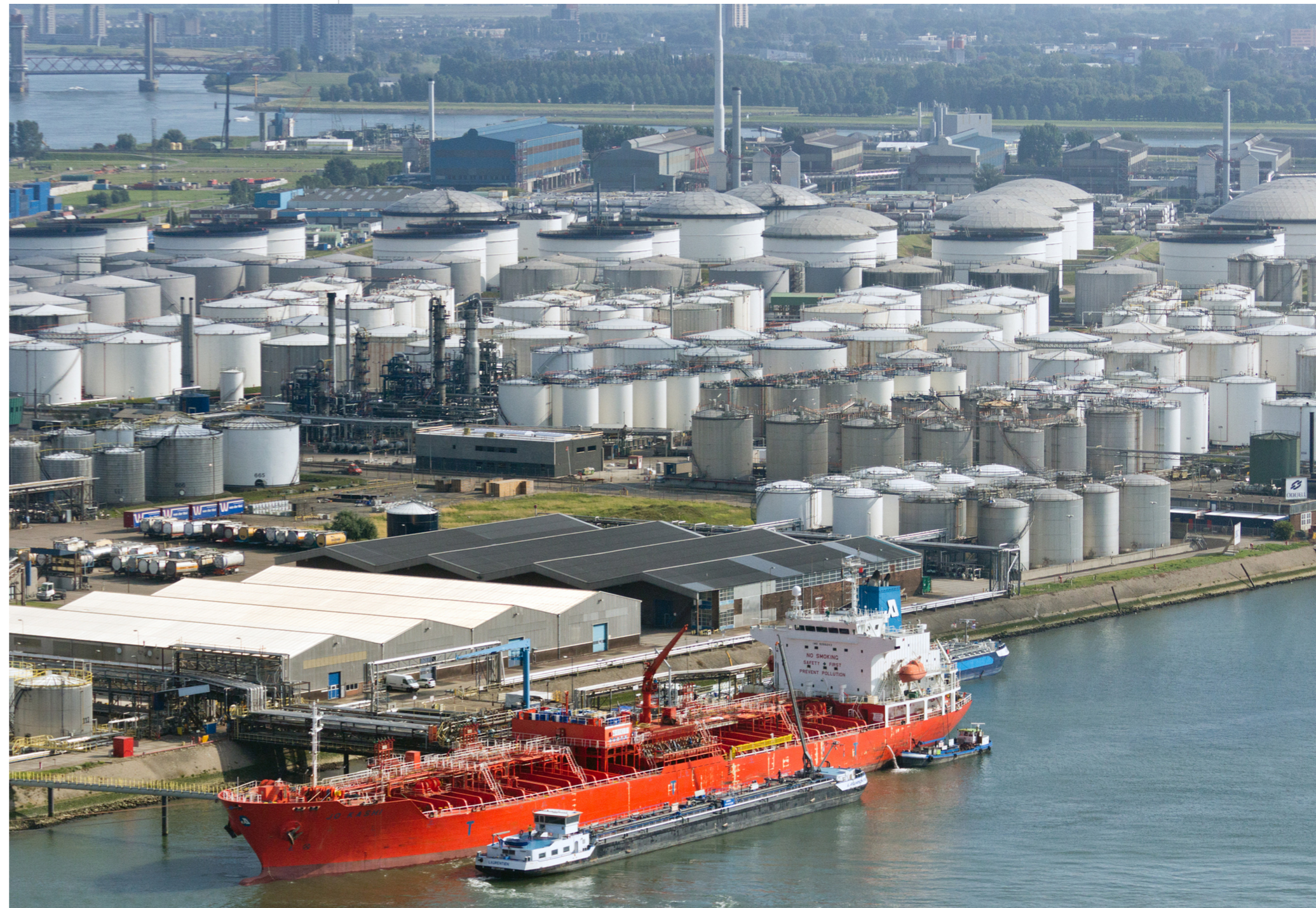
Tanker and oil storage tanks in Rotterdam, the Netherlands. Photo by VanderWolf Images/Shutterstock.
