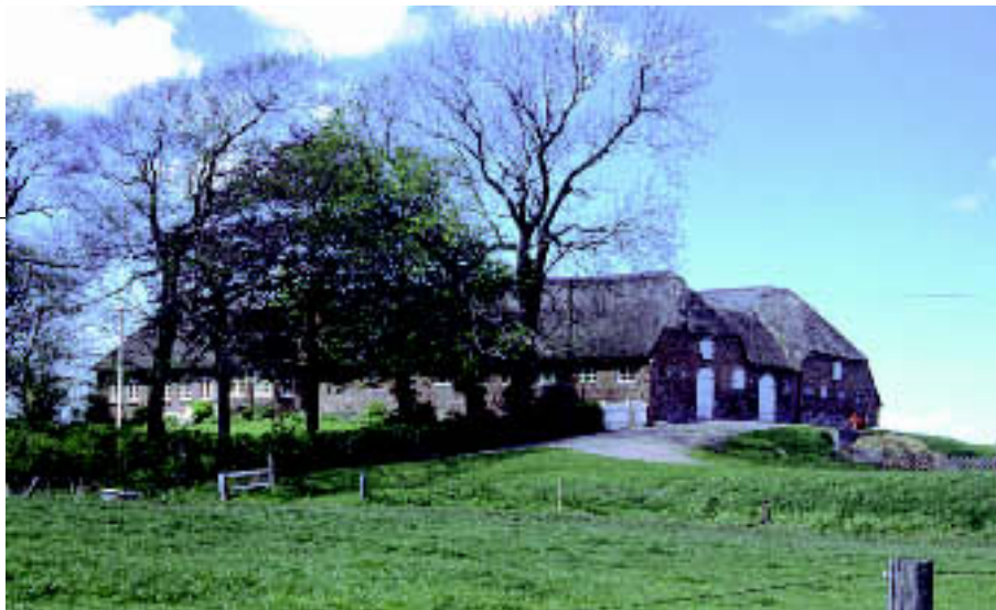
Fig. 4.19: The protected farm Sødram lies on a dwelling mound in the polder Møgeltønder Kog. It dates back to the seventeenth century and was rebuild in eighteenth century. Photo: Carl Christiansen
