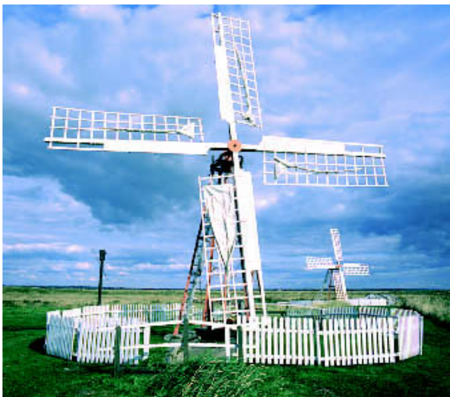
Fig. 4.17: The two pumping mills in Ballum Enge illustrate how mills were used to provide fresh water for the animals in the marsh. The mills are reconstructions built on their original place. Photo: Carl Christiansen
