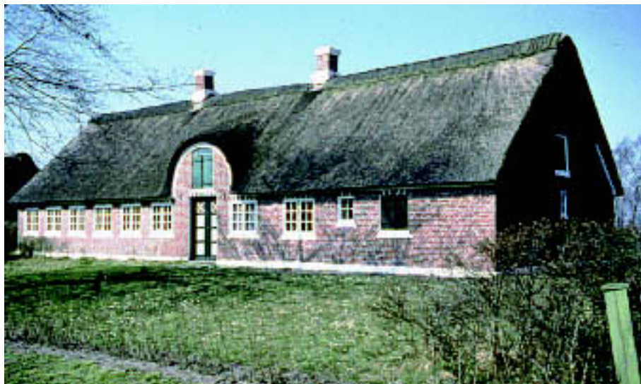
Fig. 4.27: This house from Sønderho on the island of Fanø is a typical example of a brick-built house from around 1800. Photo Steffen Søndergaard
