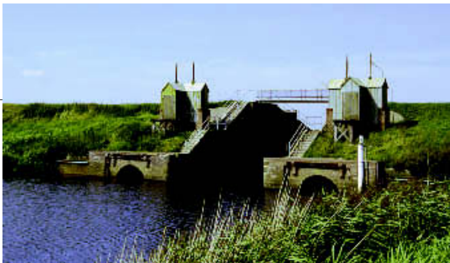
Fig. 4.22: The lock at Højer was built in 1861 and allowed ships' passage to the harbours inside the new dyke. Photo: Carl Christiansen
