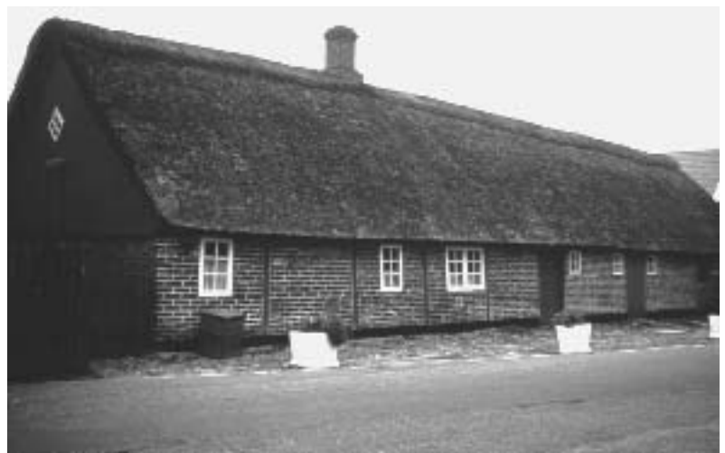
Fig. 4.7 : Timber-framed house from Nordby on the island of Fanø. It dates from the eighteenth century and represents the time before brick-building became dominant. Photo: S. Søndergaard
